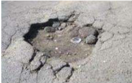
Gambar 2.15 Lubang (Potholes)
