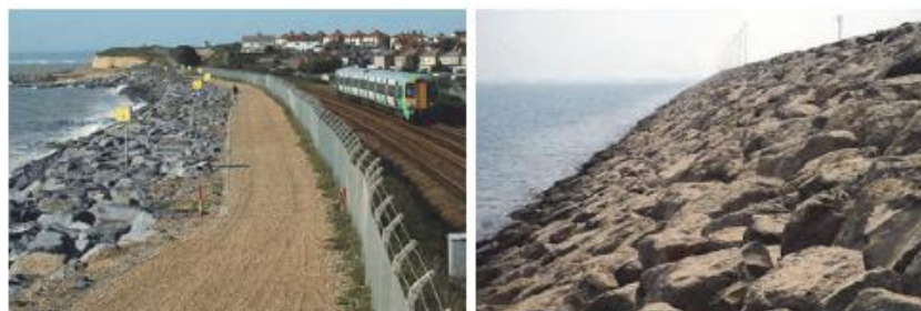
Gambar 2.7 Ruble mound Seawall (Eurotop Manual 2016)
