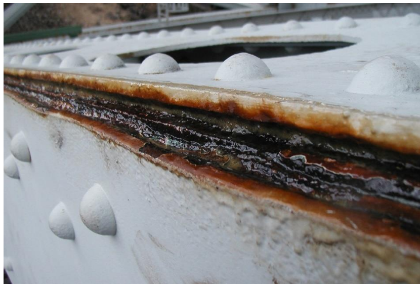
Gambar 2.7 Crevice Corrosion
