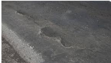
Gambar 2.14 Jembul ( upheaval )
