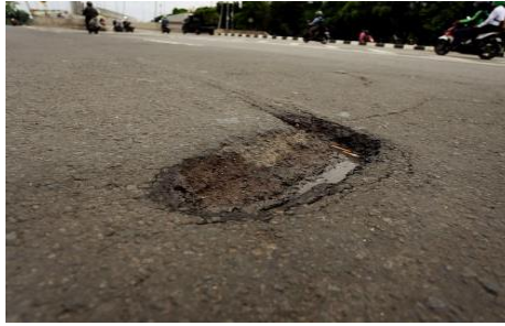
Gambar 2.15 Lubang ( potholes )
