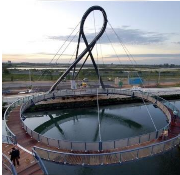
Gambar 4.20 Ponte Pedonal Circular de Aveiro https://www.skyscrapercity.com/showthread.php?t=367351
