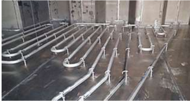
Gambar 2.15. Instalasi Pipa Heating Coil Sumber: www.koyotky.co.jp
