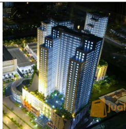
East Coast Mansion Apartment (under construction)
