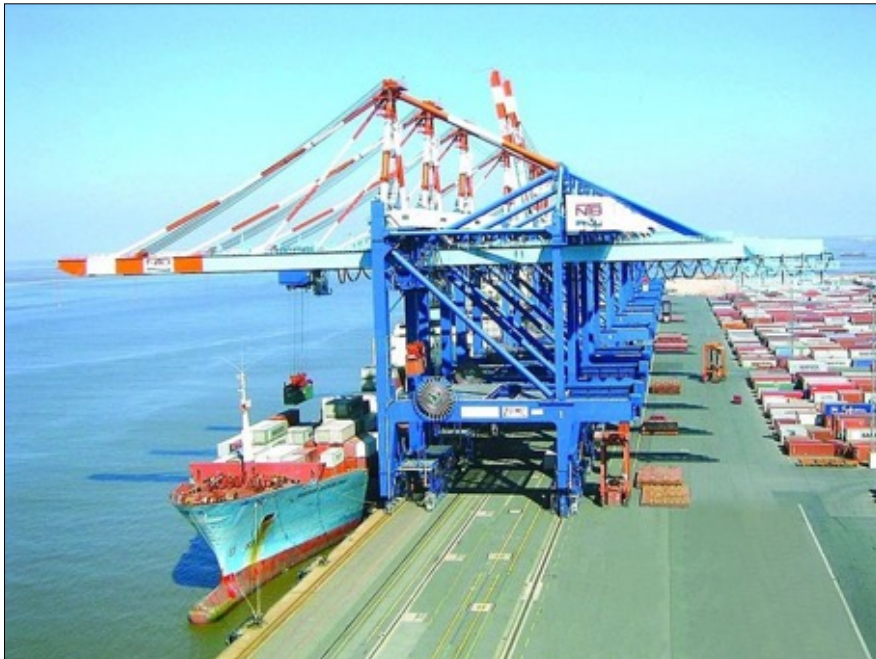
Gambar 3. 4 Post Panamax di Port Alburni, Texada Island (Sumber: www.pelindo1.co.id )
