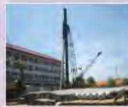
Piles Foundation for Building
