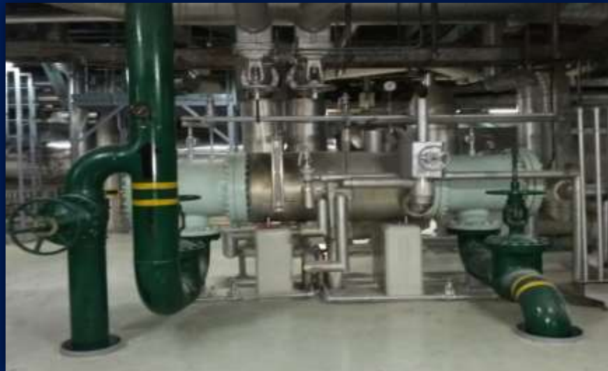
STEAM JET AIR EJECTOR
