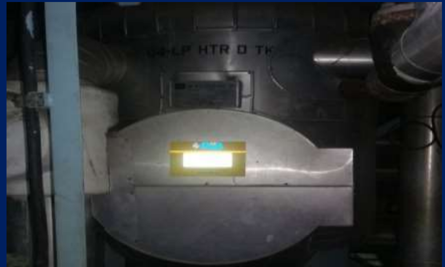
HEATER DRAIN TANK
