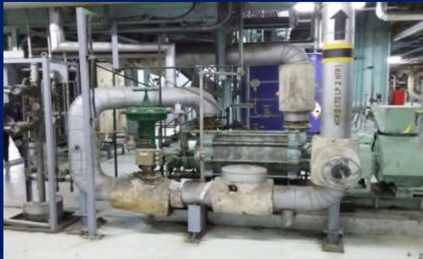
HEATER DRAIN PUMP
