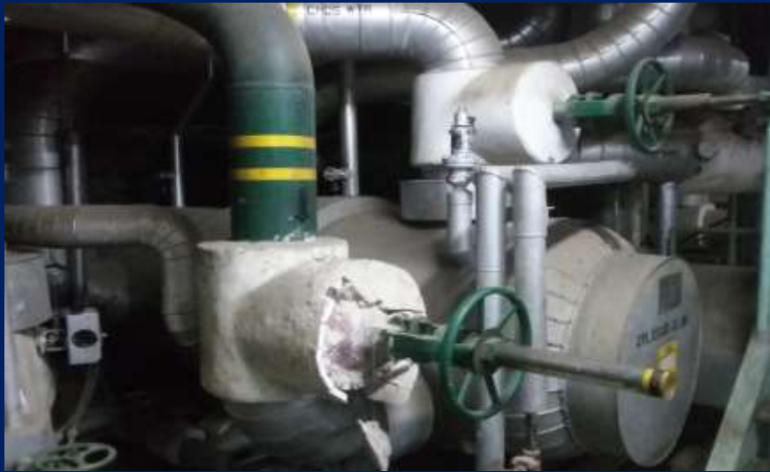
LOW PRESSURE HEATER 1
