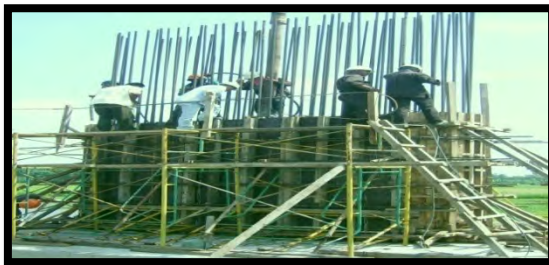
Gambar 4.7 : Pengecoran Abutment
