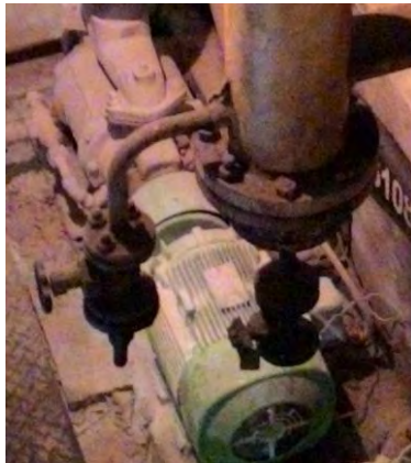
Gambar 3.3 auxilliary oil pump
