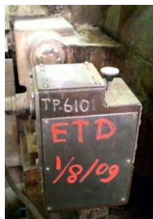
Gambar 3.5 solenoid valve
