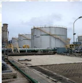
Gambar 2.7. RAW Water Tank
