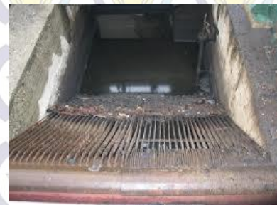
Gambar 2.2. Bar Screen (Sumber : Analisa Corrective Maintenance PT. PJB UP Gresik)
