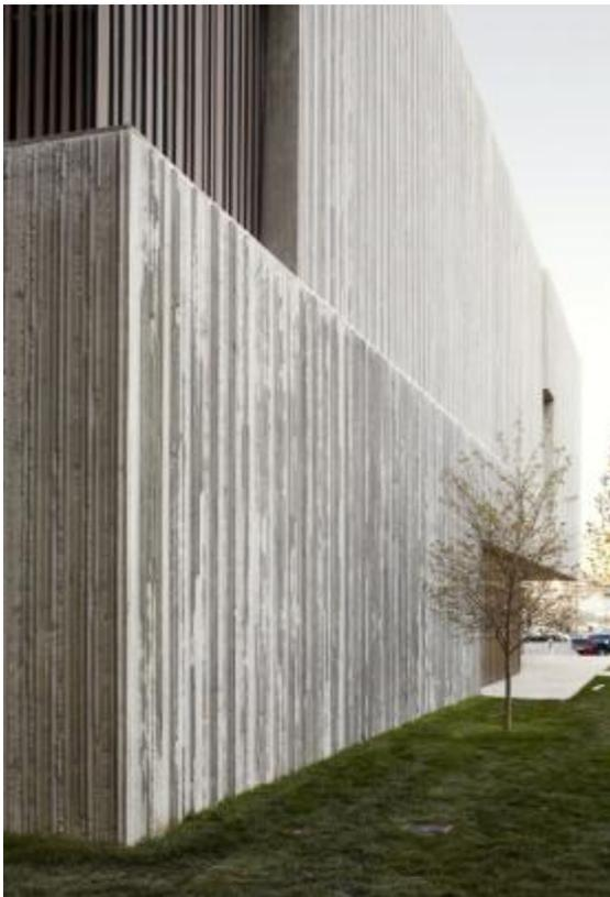
Gambar IV. 6 Material fasad GRC outdoor panel
