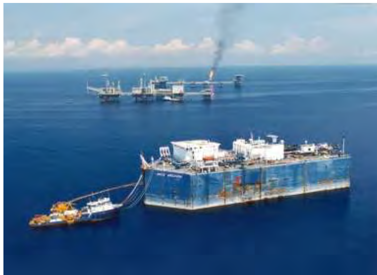
Gambar 2. 2 Floating Storage and Offloading System (FSO) (PT. PHE ONWJ, 2004)
