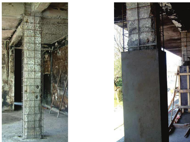
Gambar 2.2 Strengthening the column using concrete jacketing
