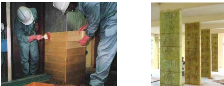
Gambar 2.6 Strengthening the column using aramid fiber reinforced polymer (sumber : https://www.researchgate.net/figure/Confining-column-with-Aramid-Fiber-sheet-JBDPA-report-2005_fig3_237841803 )
