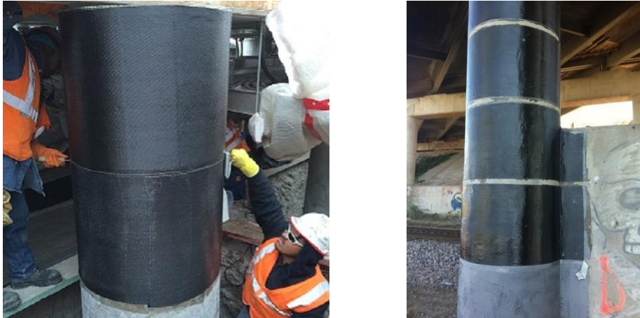
Gambar 2.4 Strengthening the column using carbon fiber reinforced polymer (sumber: http://www.materialsperformance.com/articles/material-selection-design/2016/07/gas-plant-uses-carbon-fiber-reinforced-polymer-wrap-to-strengthen-concrete-columns )
