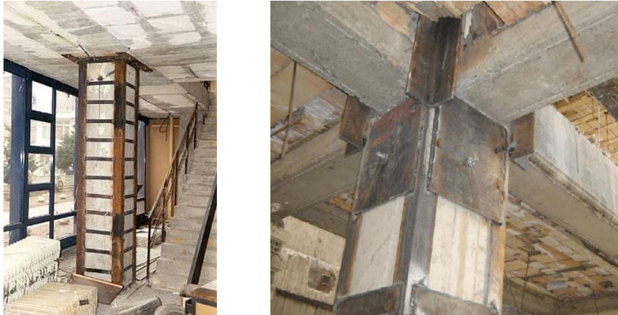
Gambar 2.3 Strengthening the column using steel jacketing
