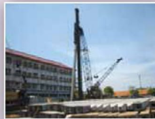
Piles Foundation for Building
