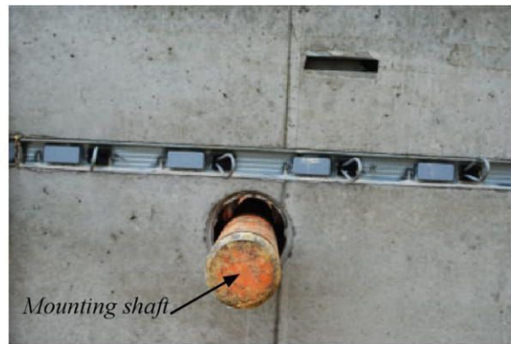
Figure 8. Mounting shaft placed in the hole.
