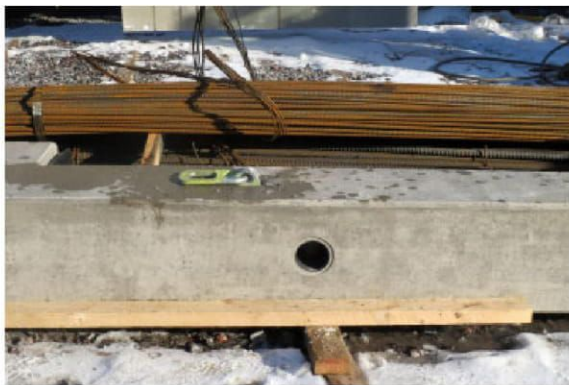
Figure 7. Hole for mounting shaft in precast element.
