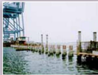
Piles for Marine Structure
