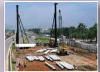
Piles Foundation for Bridges
