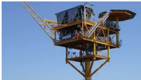
Gambar 2.1 Wellhead Platform (Sumber : Bull, 2018)
