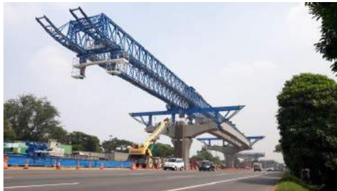
Gambar 2.10 Launcher Girder
