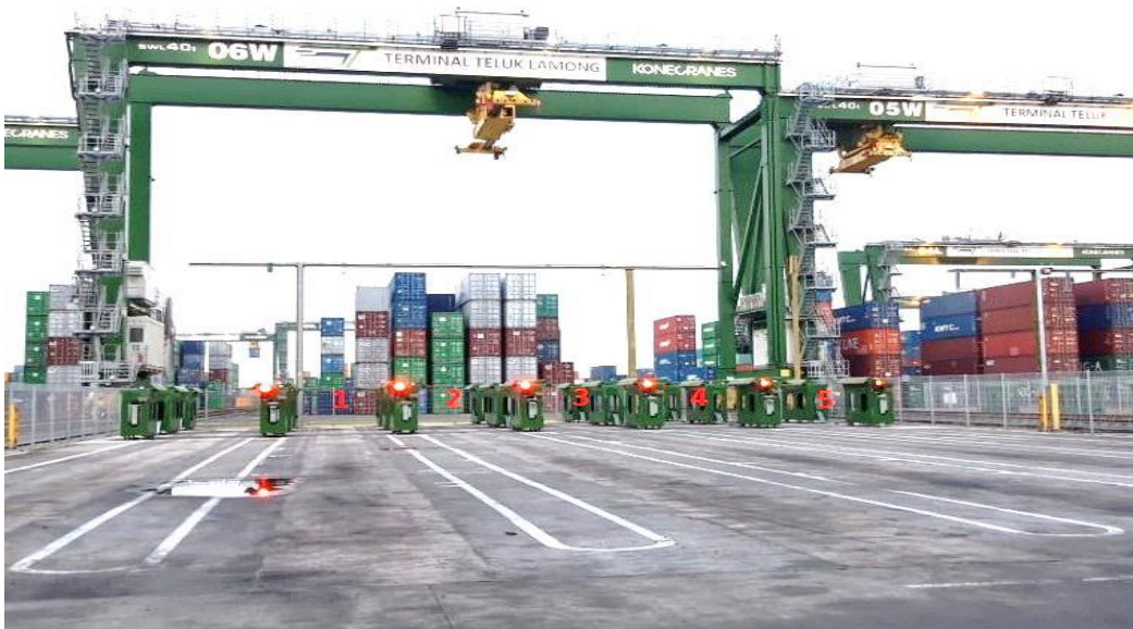
Gambar 1.2 Dock Gate di Blok Container Yard
