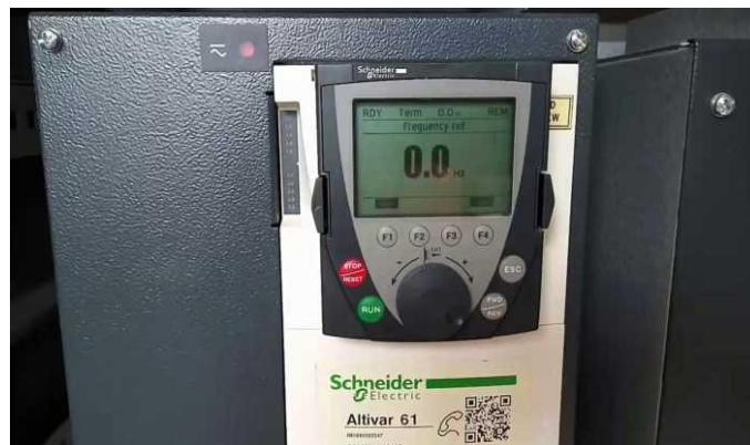
Gambar 4. 1 *Variable Speed Drive Controller*
