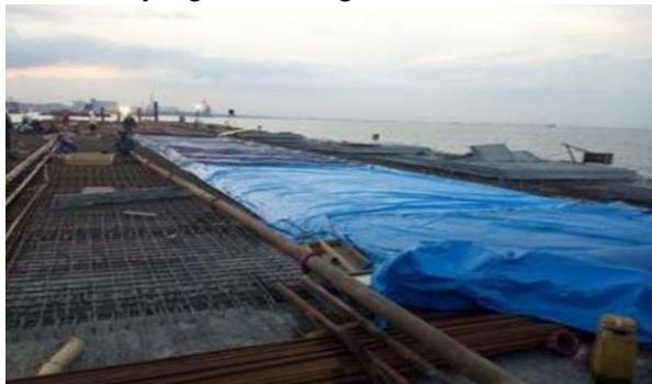
Gambar 7.50 Proses *Curing* Beton
