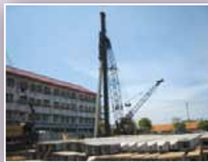
Piles Foundation for Building
