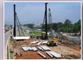
Piles Foundation for Bridges
