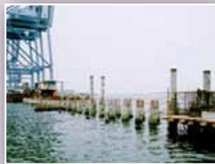
Piles for Marine Structure
