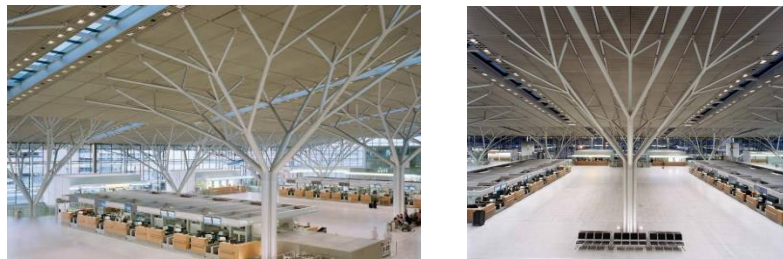
Gambar 4.9 : Struktur atap Bandara Stuttgart . Sumber : competitiononline.com
