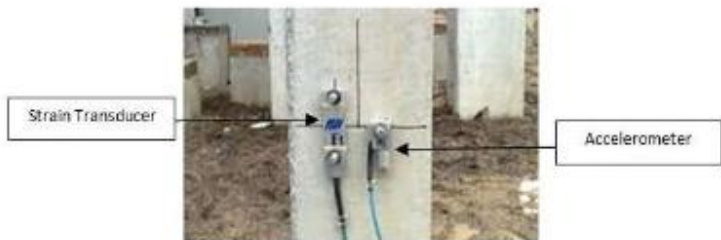
Gambar 7.20 Pemasangan strain transducer dan accelerometer
