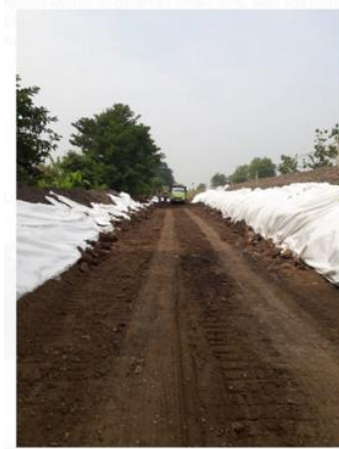
Gambar 1.4 Replacement (Sumber : Gambar Proyek)
