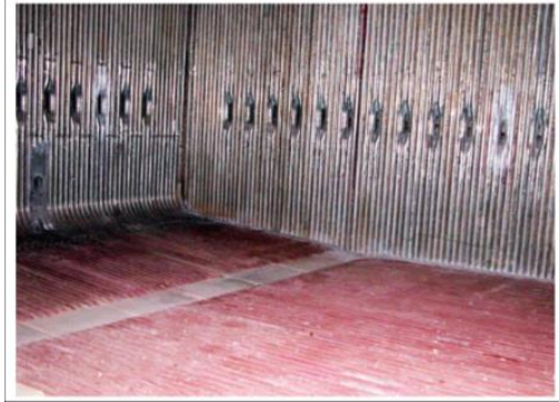
Gambar 2.10 Contoh waterwall tube
