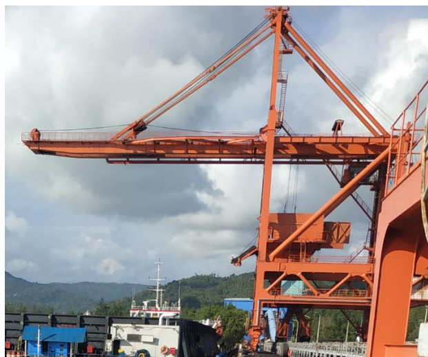
Gambar 2.15 ZQX1250 Bridge-type Grab Ship Unloader (Sumber : Penulis, 2019)
