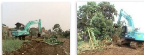
Gambar 2. 2 Clearing and Grubbing
