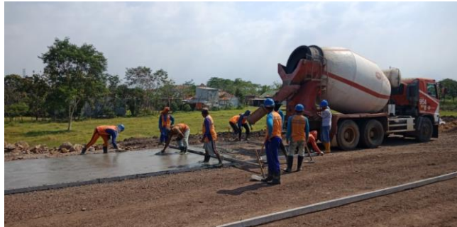
Gambar 4. 3 Proses Pengecoran Lean Concrete
