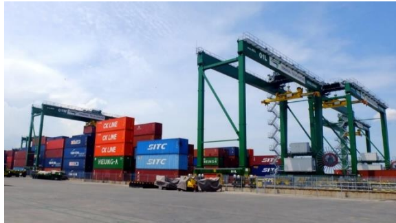
Gambar 4.4 Automated Stacking Crane (ASC)
