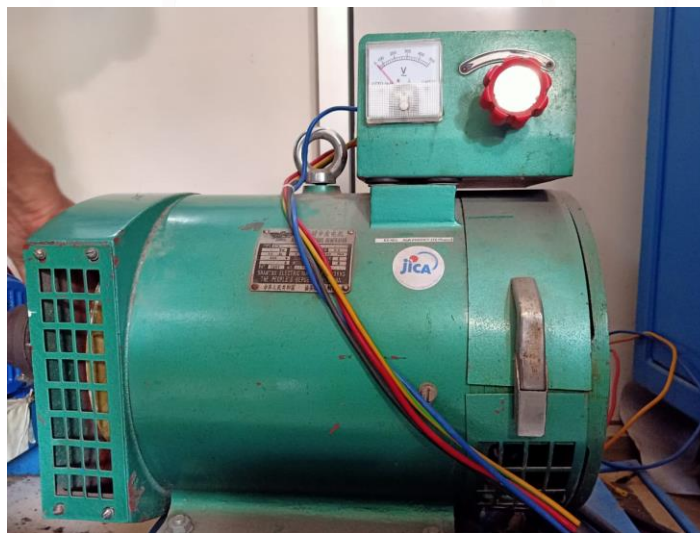
Gambar 3.4 Generator Sinkron 3 Fasa
