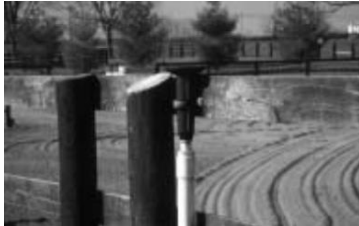
Gambar 4.16 Sprinkler lapangan kuda (Sumber: Wheeler, Eileen. 2006. Horse stable and riding arena design. Blackwell Publishing)
