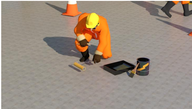
Gambar 8.14 Ilustrasi pengolesan corrosion inhibitor
