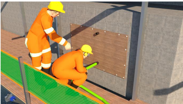
Gambar 8.36 Ilustrasi Proses Injection Grouting Non-Shrink
