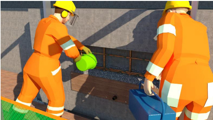
Gambar 8.34 Ilustrasi Pre-Placed Aggregate
