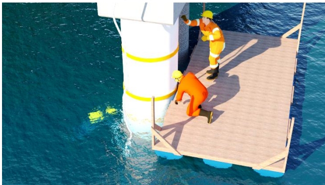
Gambar 8.47 Ilustrasi proses injeksi epoxy grout
