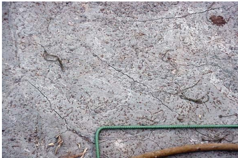
Gambar 2.8 Thermal cracks in a thick slab (Sumber: CTL, 2002)
