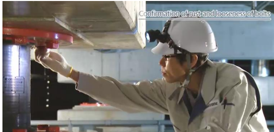
Gambar 10. 18 Pengecekan Karat dan Baut (Bridgestone, 2013)
