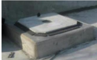
Gambar 10. 9 Grouting base plate
