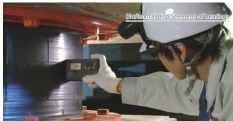
Gambar 10. 19 Pengecekan perpindahan horisontal (Bridgestone, 2013)
