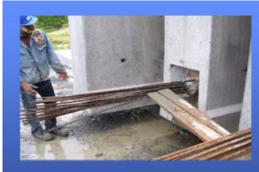
Gambar 4. 36 Stressing Length Dipotong
