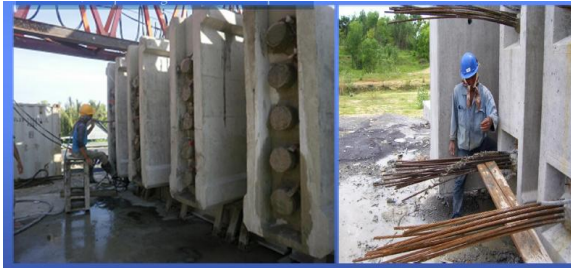
Gambar 4. 34 Mortar Grouting Dipompa Kedalam Tendon
