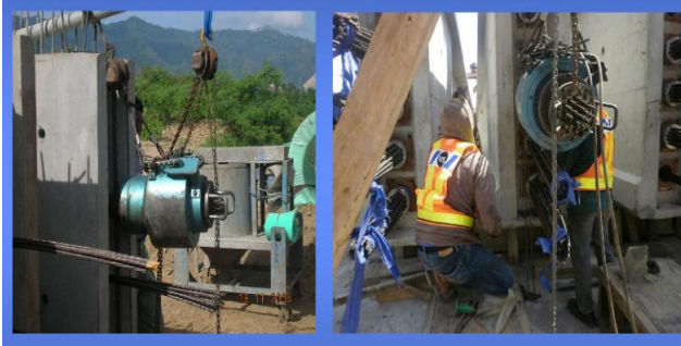
Gambar 4. 14Pemasangan Hydraulic Jack
