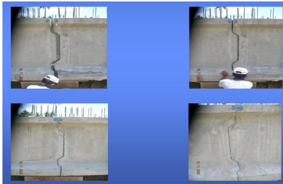
Gambar 4. 17Perapatan Segment Girder
