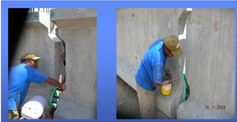
Gambar 4. 16Mengoleskan Epoxy
