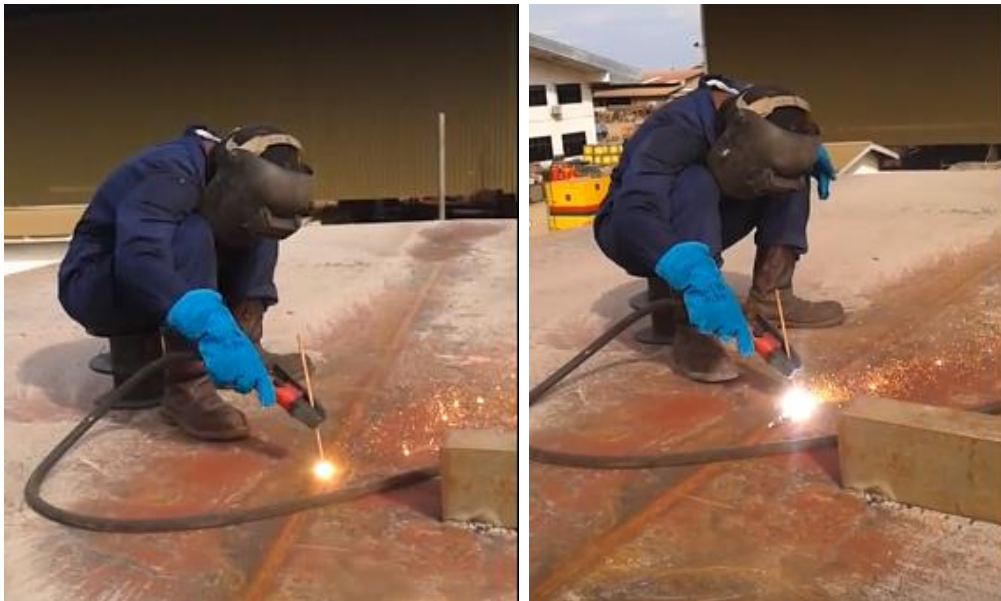
Gambar 4.5. Repair Goughing
