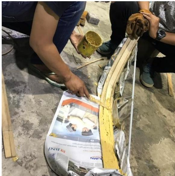
Gambar 4.12 Proses Laminasi Gading Bambu
