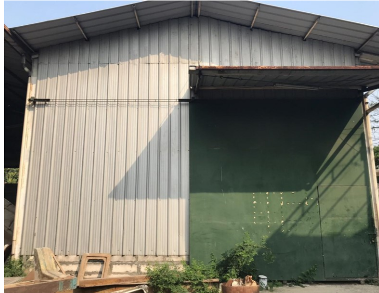
Gambar 4.11 Gudang material galangan PT. Royal Advance Fiber
