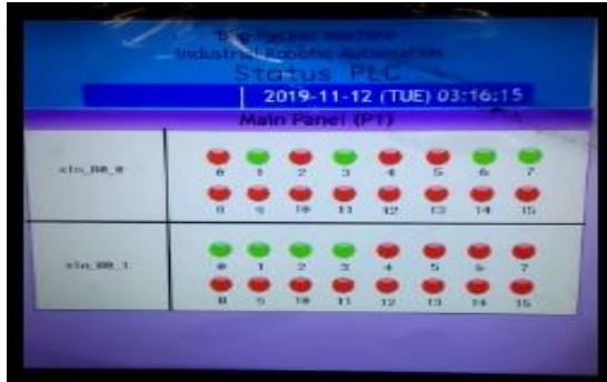
Gambar 4. 1 Status PLC (P1) Main Panel
