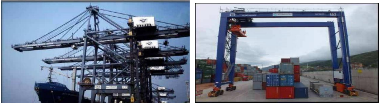
Gambar 2. 3 Quay Container Crane dan Rubber Tyre Gantry Crane
