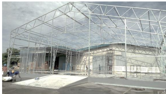
Gambar 2. 25 Rangka Aluminium (Sumber: Ghazali, 2018)
