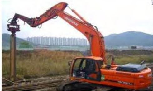
Gambar 2.4 Vibrator pile driver
