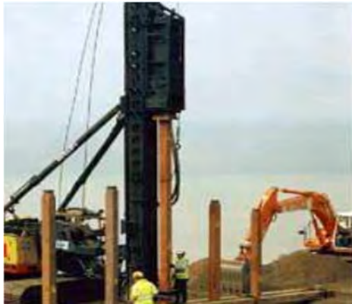
Gambar 2.2 Drop Hammer
