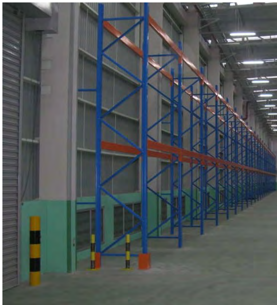
Gambar 4.2. Racking SPR (Single Pallet Rack)
