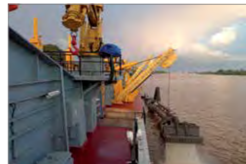
TRAILING SUCTION PIPE IN GANGWAY
