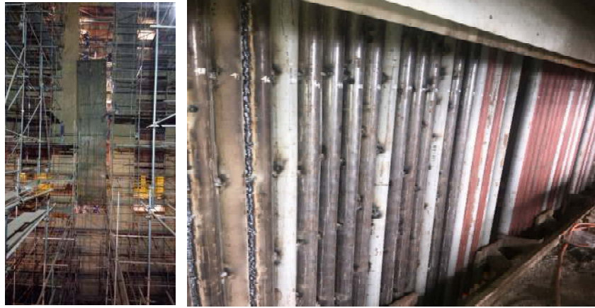
Gambar 2.4 waterwall tube boiler
