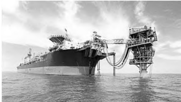
Gambar 2.8 Fixed Tower (Sumber: Helmidadang, 2012)
