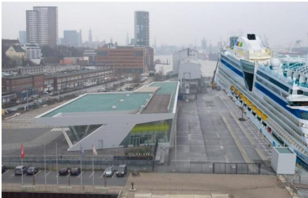
Figure 0-1 Electric shore power at the cruise terminal Altona
