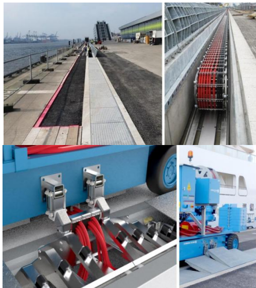
Figure 0-12 Cable duct and cover lifting device with cable guideway
