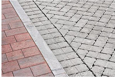
Gambar 2.3 Jalan Paving Block
