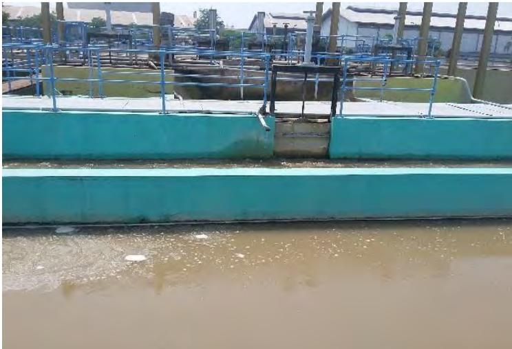
**Gambar Unit Flokulasi IPAM Karang Pilang I**
