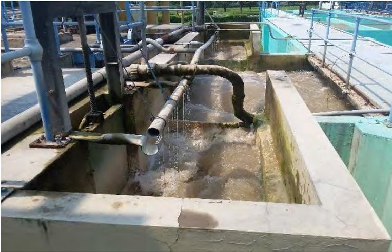
**Gambar Unit Koagulasi IPAM Karang Pilang I**
