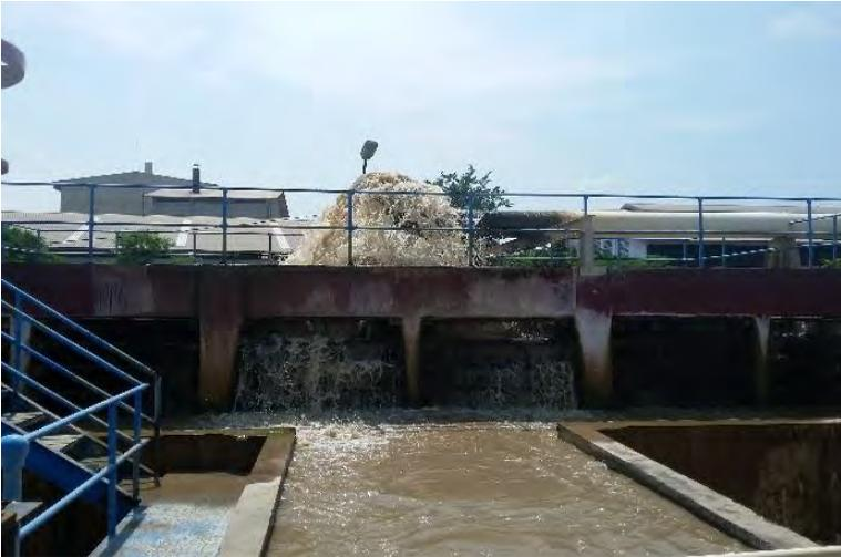
**Gambar Unit Aerasi IPAM Karang Pilang**
