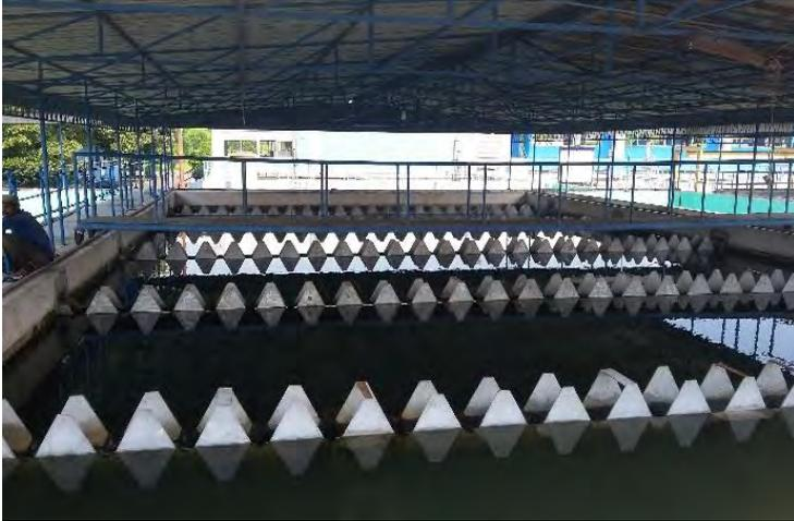
**Gambar Unit Clarifier IPAM Karang Pilang I**
