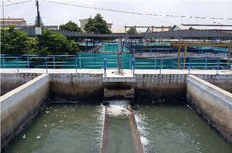
**Gambar Unit Filter IPAM Karang Pilang I**
